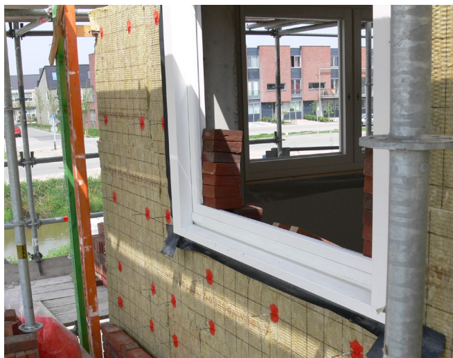
Prikspouwanker met UNI-CLIP
